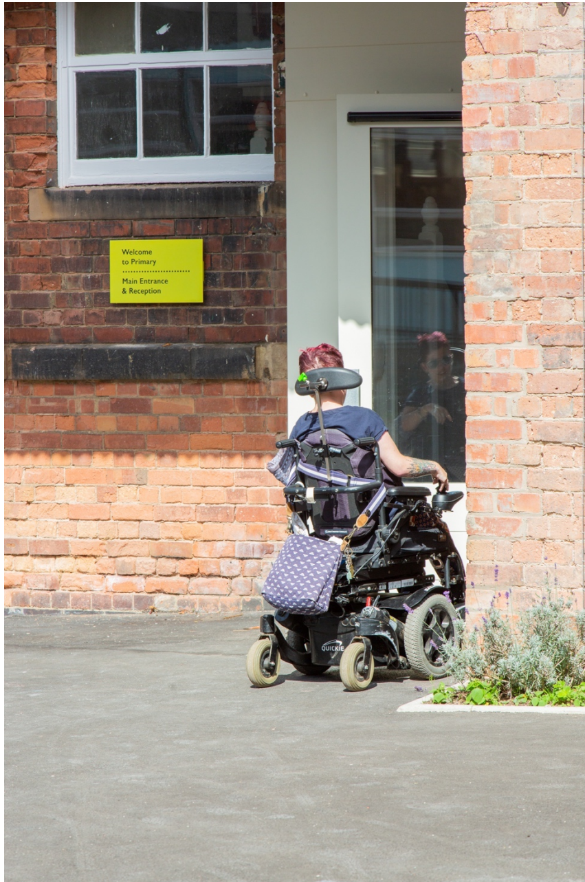
The main entrance to the building is the white door under the canopy.
